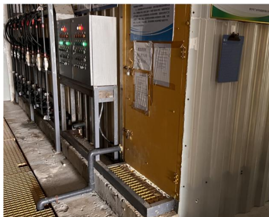
储酸间收集槽
